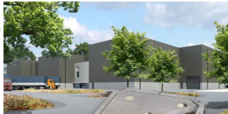
Installation for the production of monoliths (IPM)
