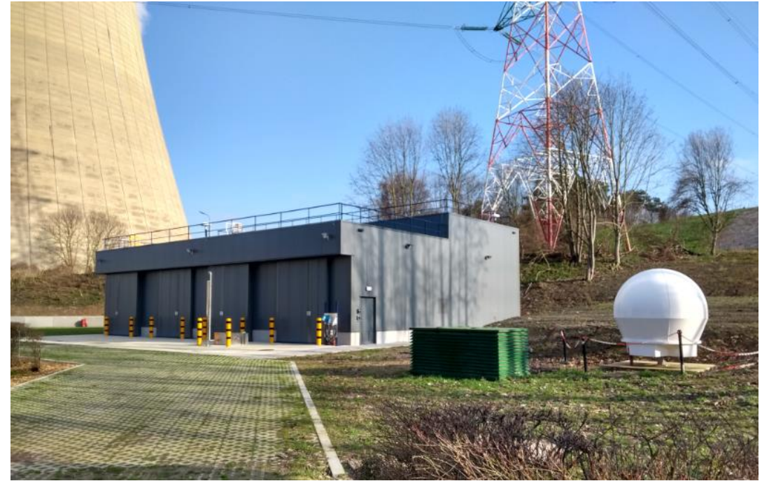
New back-up crisis centre building
