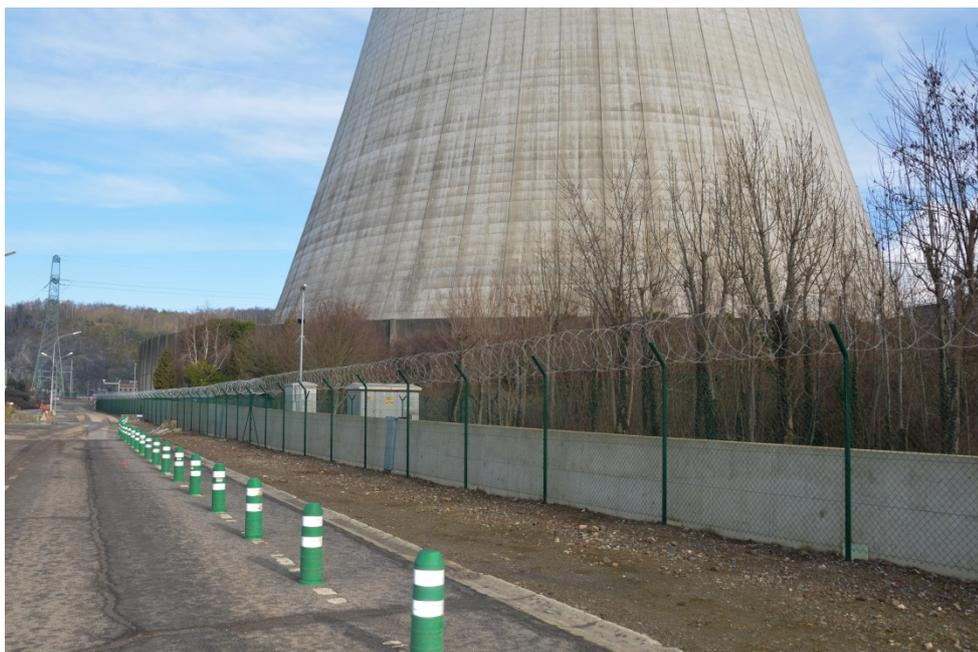
Figure 2: Peripheral protection of the site of Tihange against beyond-design flooding
